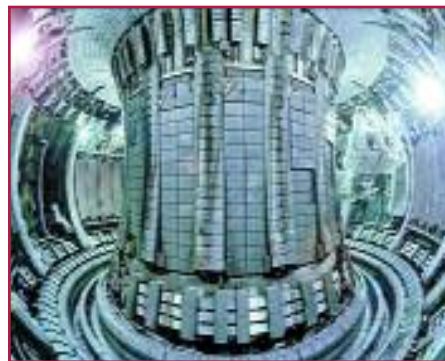
View of inside the JET Torus
