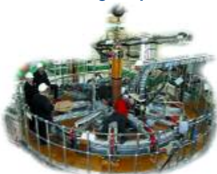
Installation of new MAST centre column
