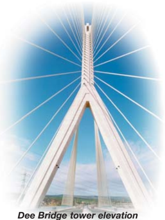
Dee Bridge tower elevation
