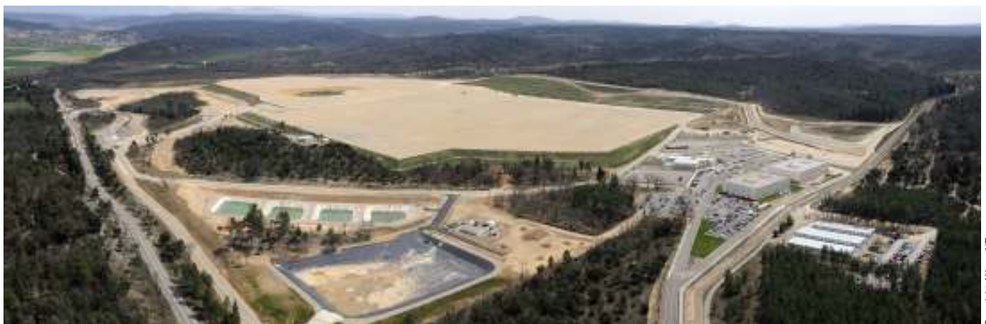
Looking north-east over the ITER construction site.
